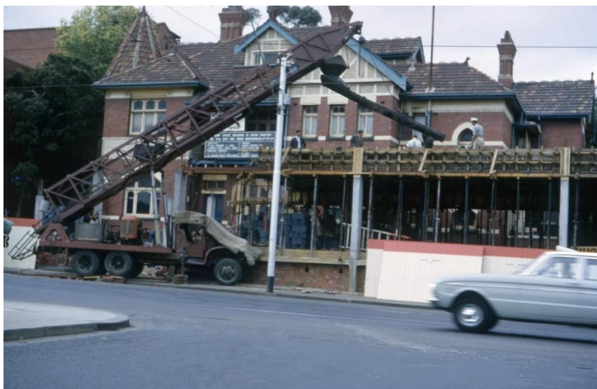
1965: A Bond concrete hoist truck at a High St., Prahran work site
